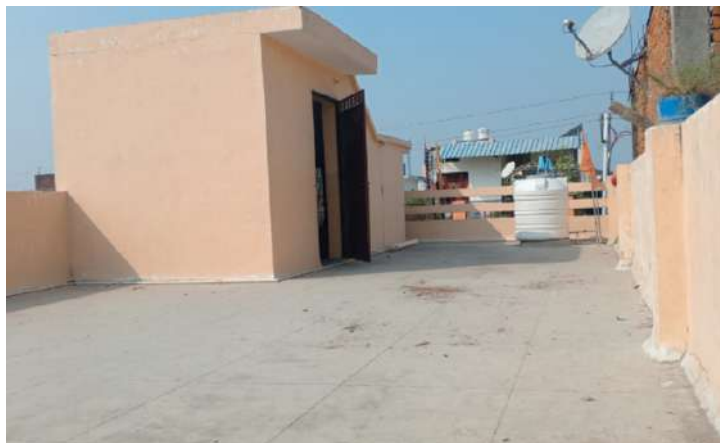
Sanction School Roof Renovation
